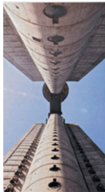
Mihajlo Mitrović, Genex Center Building, detail, Novi Beograd, 1970–1980.
